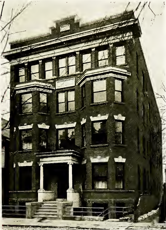
The Burdick Apartment House West Union Street
